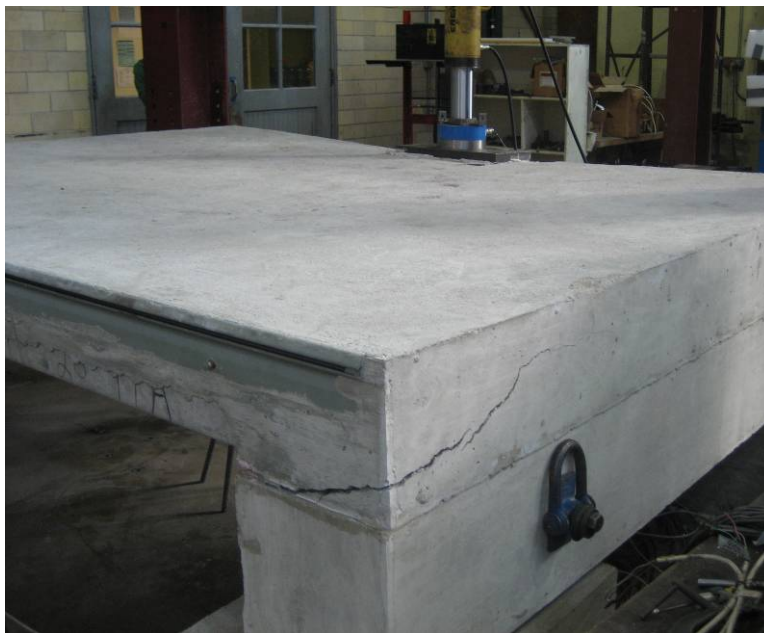
Figure 5.18: Delamination from Support Beams at Northeast Corner of Specimen P0P2
