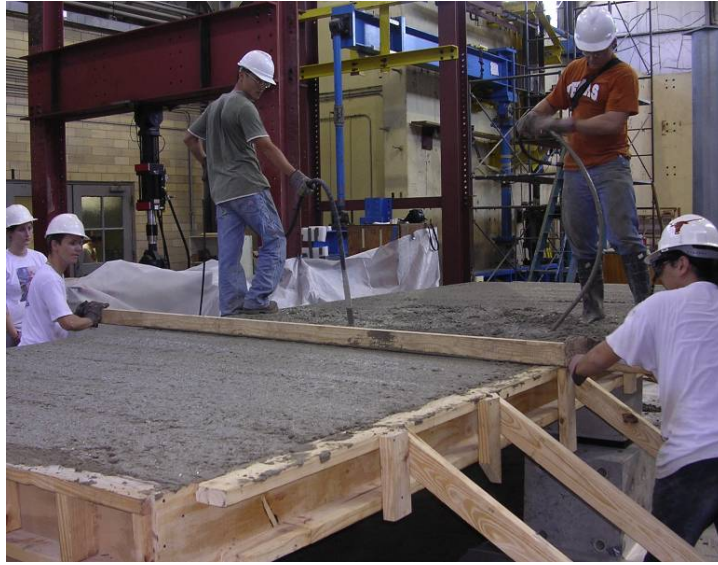
Figure 4.12: Placing Topping Slab on Specimen NOP1
