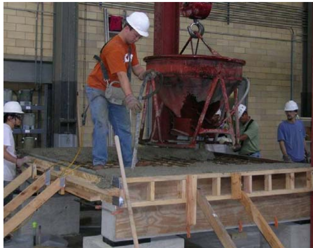
Figure 4.7: Placing Topping Slab for Specimen POP1
