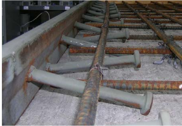
Figure 3.26: SEJ-A Steel Studs Prior to Casting
