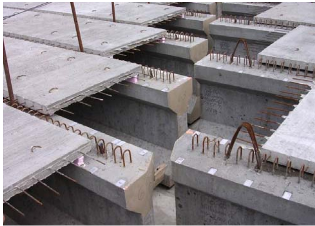
Figure 1.6: Construction of Expansion Joint with Skewed Angle Orientation
