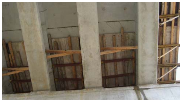
Figure 1.5: View from Underneath Bridge of Formwork for IBTS Detail
