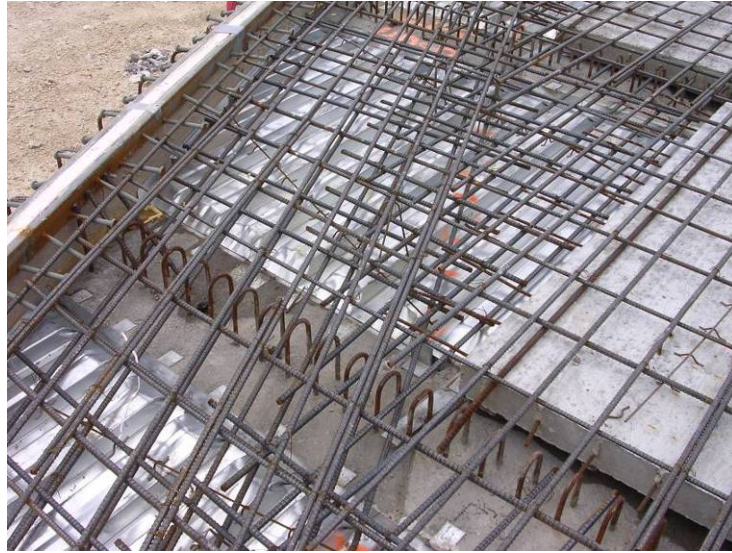
Figure 1.7: IBTS Detail Prior to Casting Topping Slab
