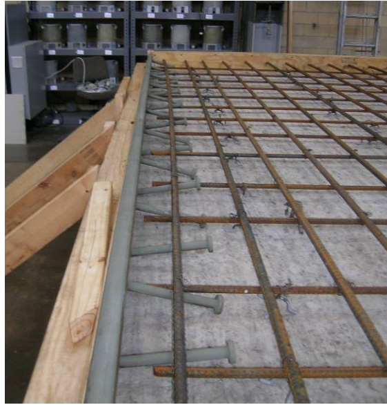
Figure 4.4: SEJ and Reinforcing Steel Prior to Casting Topping Slab
