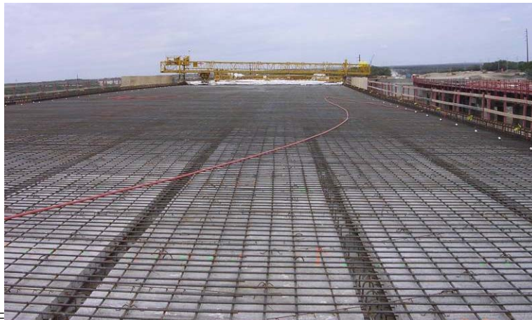
Figure 1.3: PC Panels and Reinforcing Steel Prior to Casting Topping Slab
