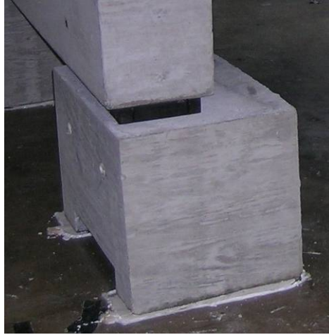
Figure 3.19: Concrete Support Block and Bearing Pad
